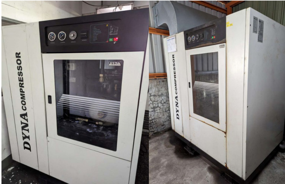
Replacement of obsolescent air compressors to increase power by nearly 14%
